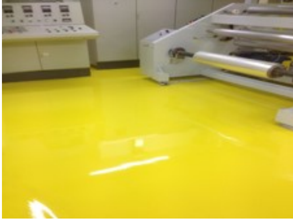
Manufacturing Facility - Installed by IFT
