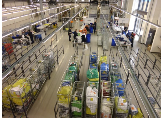
Laundry Facility - Installed by IFT
